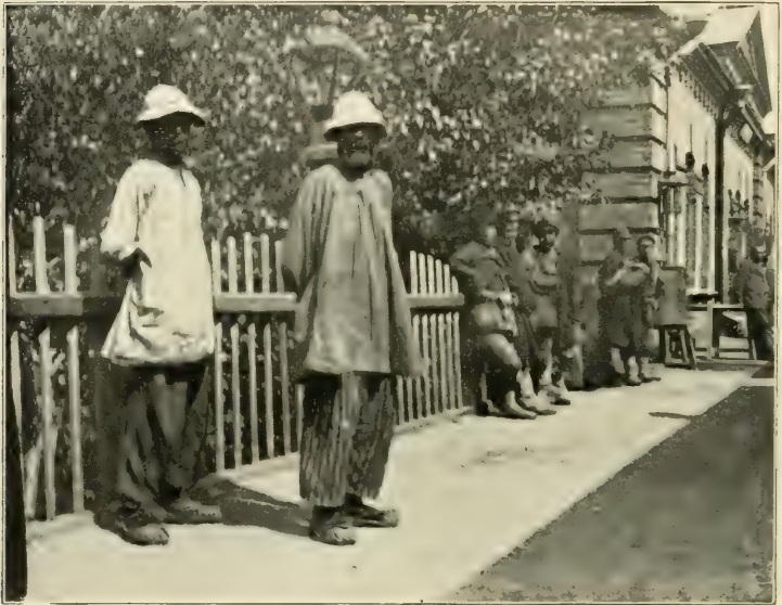
STATION ON TRANS-CASPIAN RAILWAY
